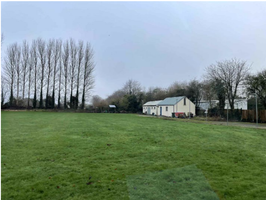
OPEN SITE AREAS TO REAR, SCOUT STORAGE BUILDINGS
